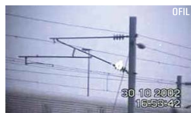
OH catenary Corona insulator
