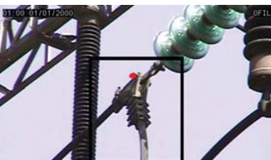
In transmission Corona on recloser
